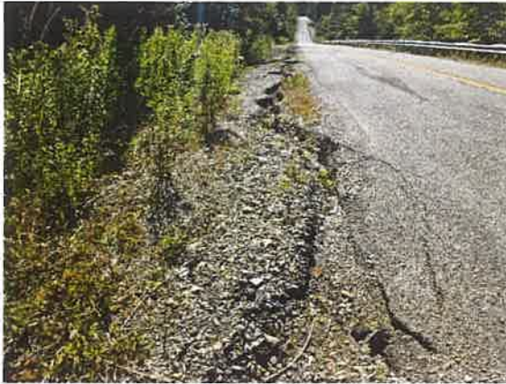
Photo 1: Shoulder damage at Civic 3999
