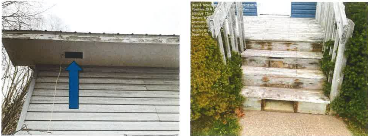
Figure 5. Left: Openings on the roof of the Alma Fire Department are susceptible to ember penetration. Right: Wooden steps with gaps and openings are located between two coniferous hedges, creating a potential vulnerability to fire spread.
