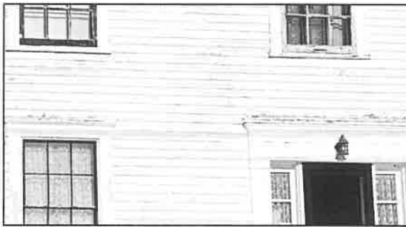
Figure 50: Detail of visible paint deterioration at front of house
