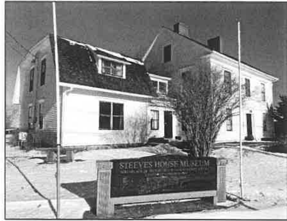
Figure 32: Current exterior documentation
