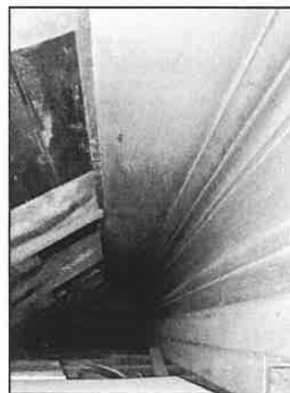
Figure 42: c.1840 exterior wall seen through hatch north of main attic
