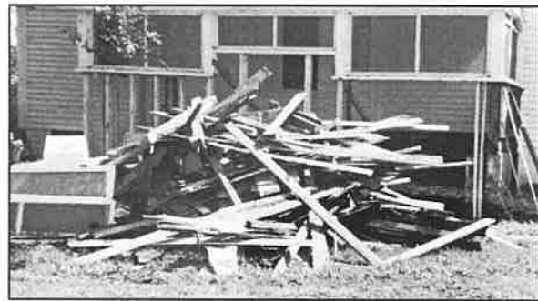
Figure 7: Historic photo showing extent of above-ground work done in 1983; note that the porch foundation was completely rebuilt at that time
