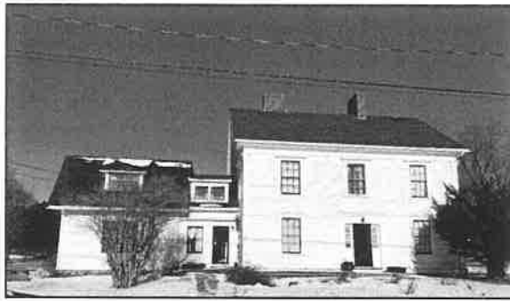
Figure 33: Current exterior documentation
