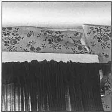
Figure 74: Above north window on east wall of the Cabin
