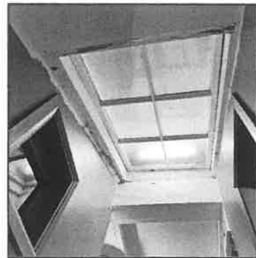
Figure 76: Detail of second floor skylight
