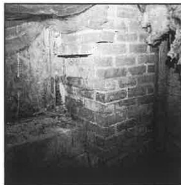
Figure 90: Base of chimney that no longer exists
