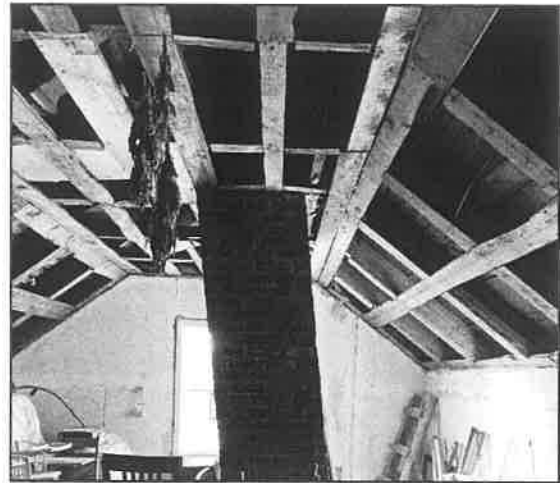
Figure 4: Simple roof structure seen in the attic
