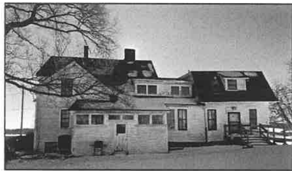
Figure 34: Current exterior documentation
