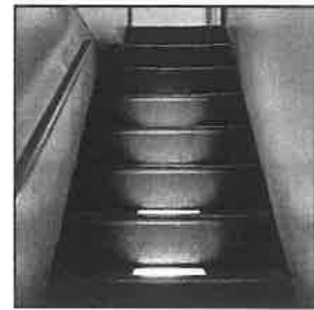
Figure 37: Servants' stair showing light through glass prism inlays
