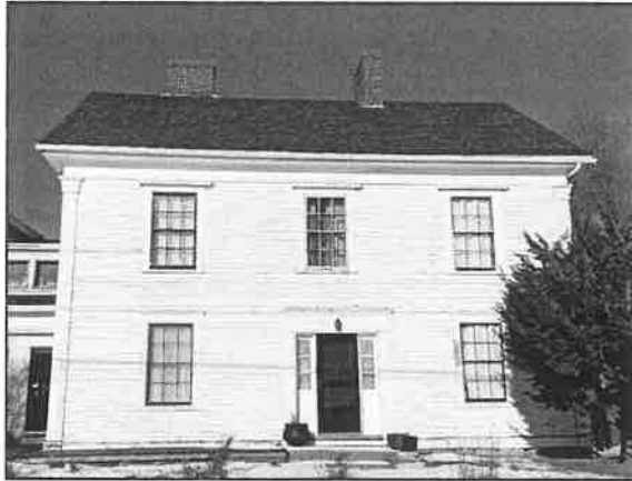
Figure 43: The two chimney stacks, the angled chimney is the one on the left (west)
