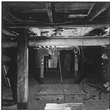
Figure 83: Looking west towards Barn addition, note the poured concrete floor
