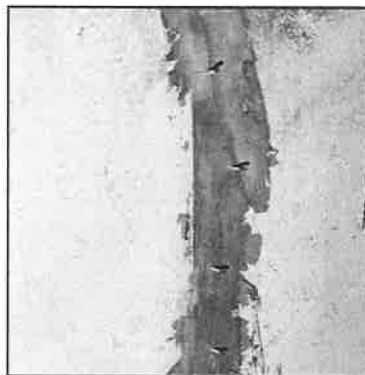
Figure 84: Concrete crack repaired with injection-based techniques
