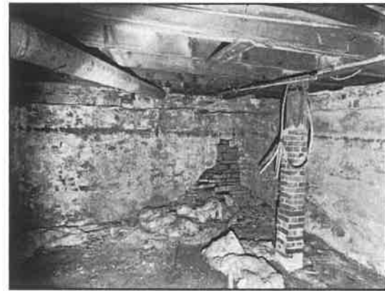
Figure 8: Basement where walls are visible
