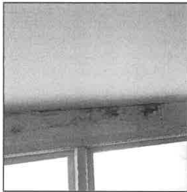
Figure 75: Above exterior porch door
