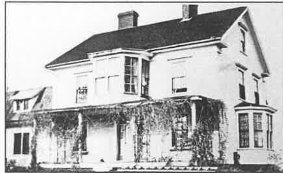
Figure 28: Ca. 1920, with front porch and bay windows still intact; the Egypt room addition is visible on the left
