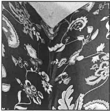
Figure 60: Moisture damage in front entry to the right of the door
